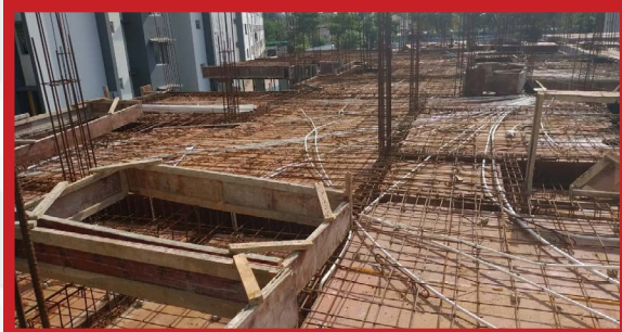
BLOCK B – 2 nd Floor Slab Electrical Conduit Work in Progress
