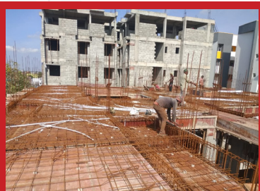
BLOCK B – 2 nd Floor Slab Electrical Conduit Work in Progress
