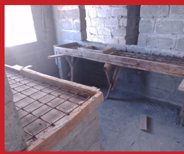
BLOCK C – 2 nd Floor Kitchen Platform Work in Progress
