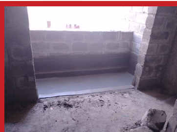
BLOCK C – 1 st Floor Balcony Waterproof Work in Progress
