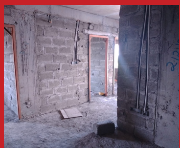
BLOCK C – 2 nd & 3 rd Floor Electrical Work in Progress
