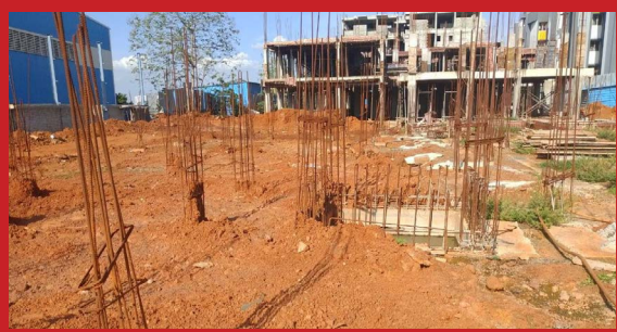
BLOCK A – Plinth Beam PCC & Shuttering Work in Progress
