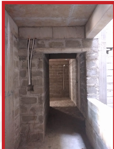
BLOCK C – 2 nd & 3 rd Floor Electrical Work in Progress
