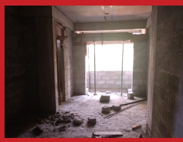
BLOCK D – 1 st Floor Lintel & Sunshade Shuttering Work in Progress
