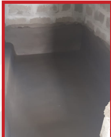
BLOCK C – 1 st Floor Toilet Sunken Waterproof Work in Progress
