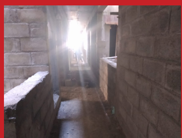
BLOCK D – 1 st Floor Block Work in Progress
