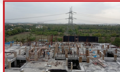
Block C - Head room shuttering work in progress
