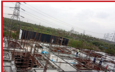
Block B - 4 th floor slab completed
