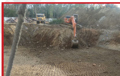
Block J and Block K - Excavation completed
