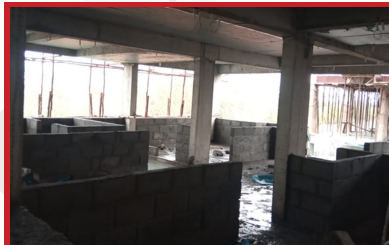
Block C - 3 rd floor block work in progress
