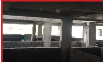
Block B - 1 st floor block work in progress
