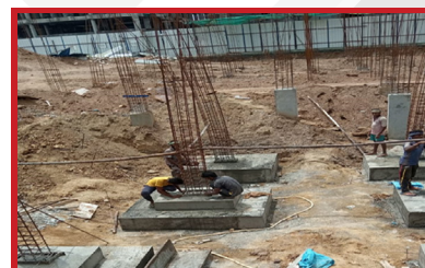
Block J - Footing work completed
