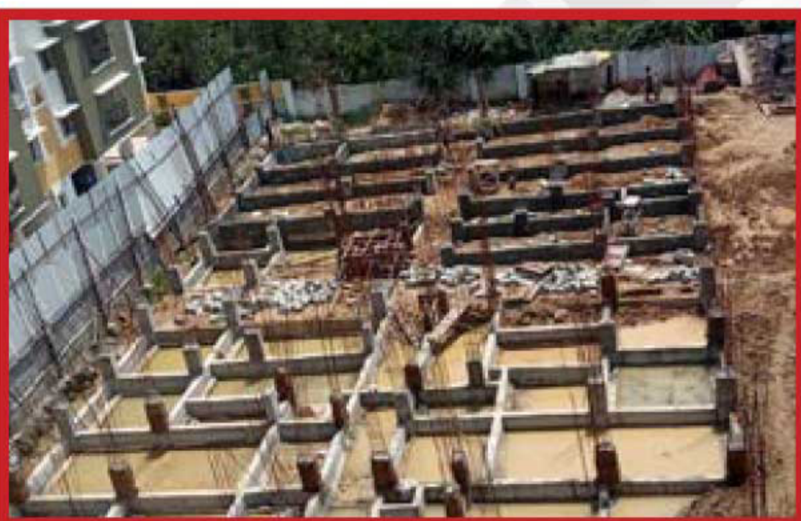
Block J - Plinth Beam: Concreting completed
