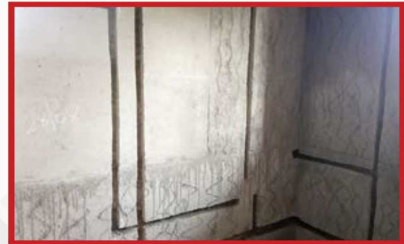
Block C - 1 st Floor: Plumbing work in progress
