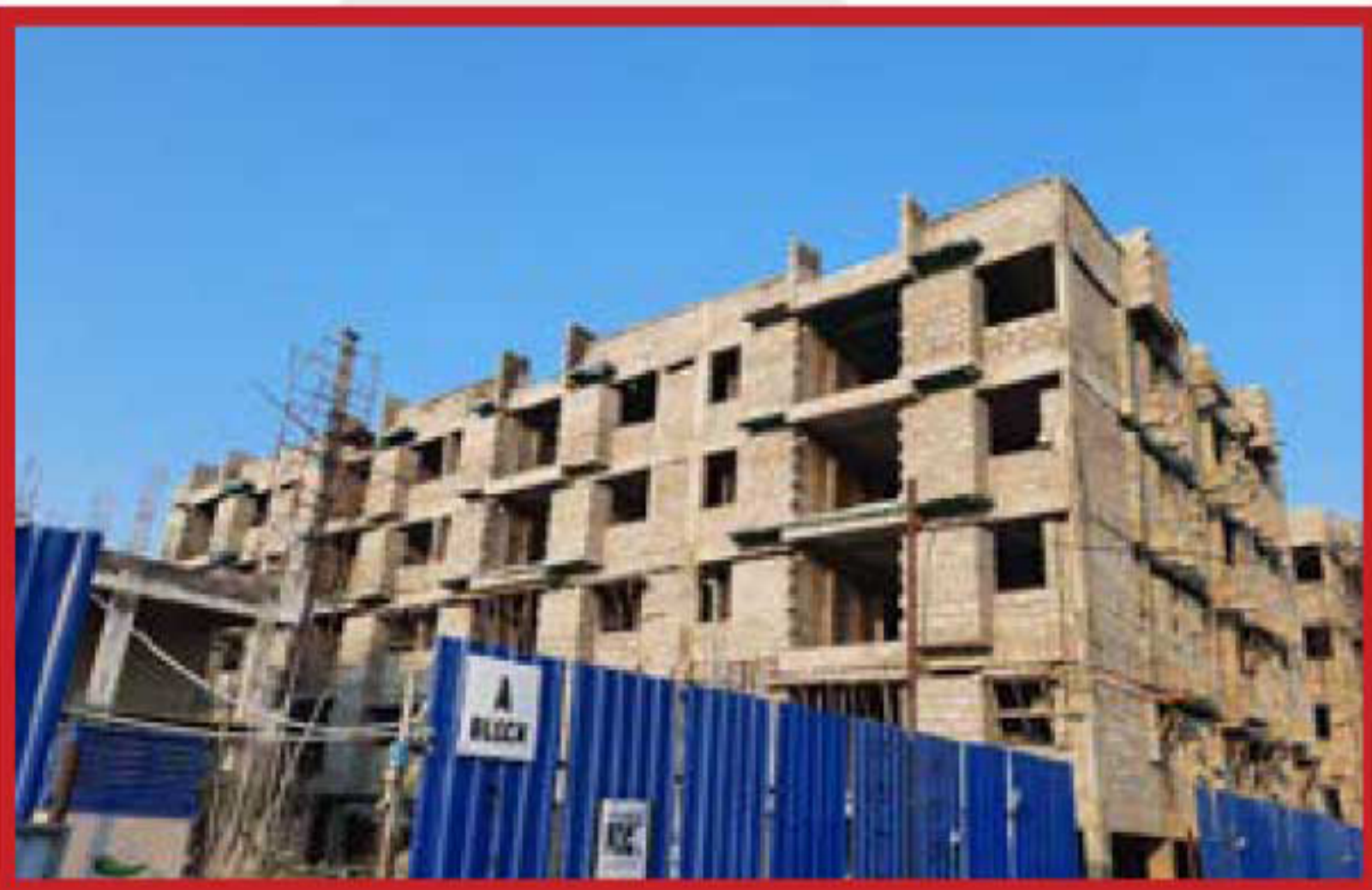
Block B - Block work completed
