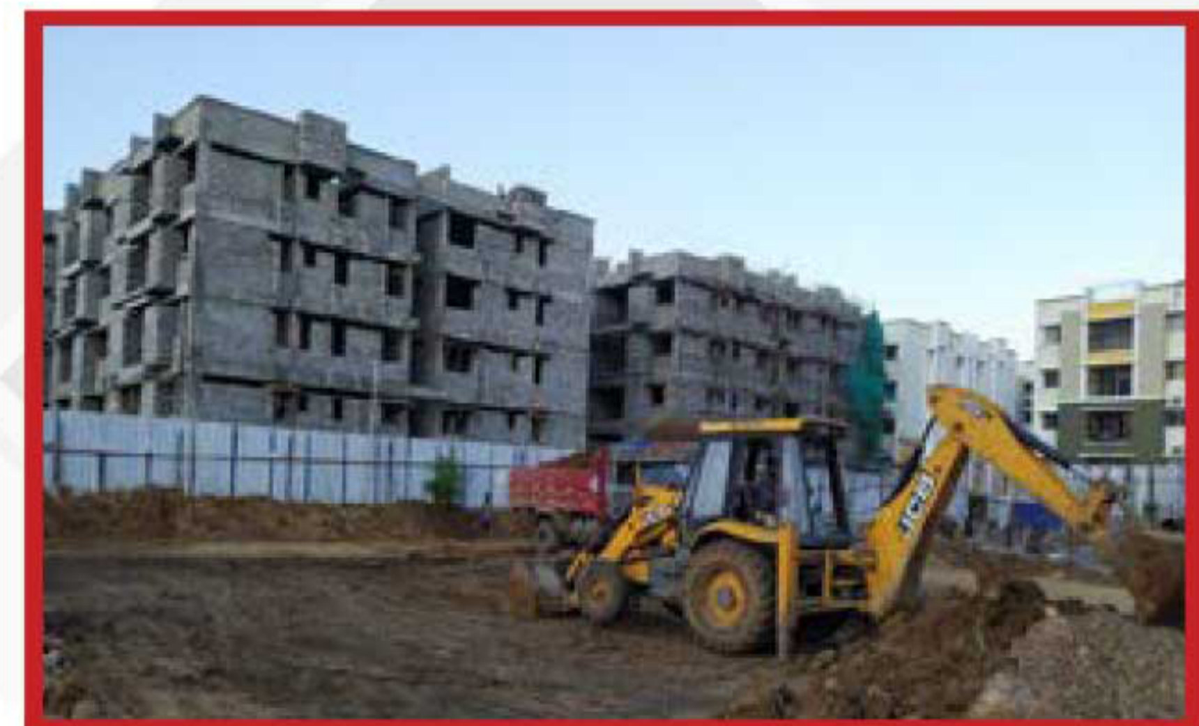
Block K - Foundation excavation in progress
