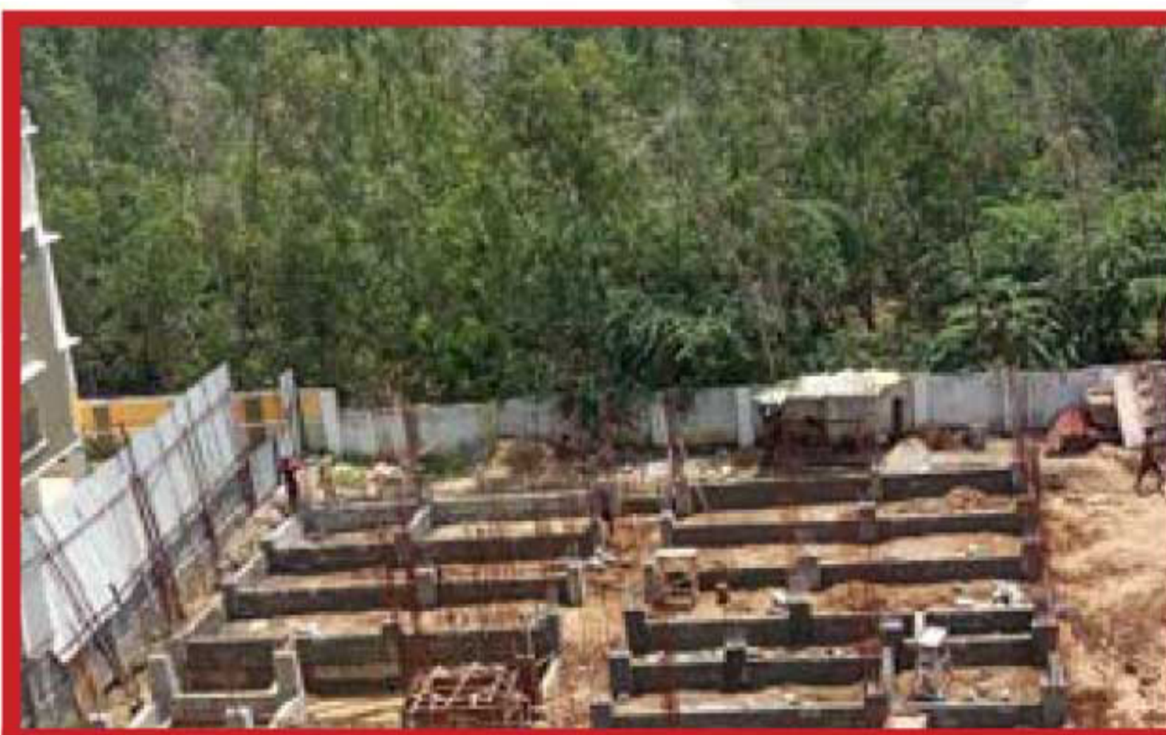
Block J - Soil refilling in progress
