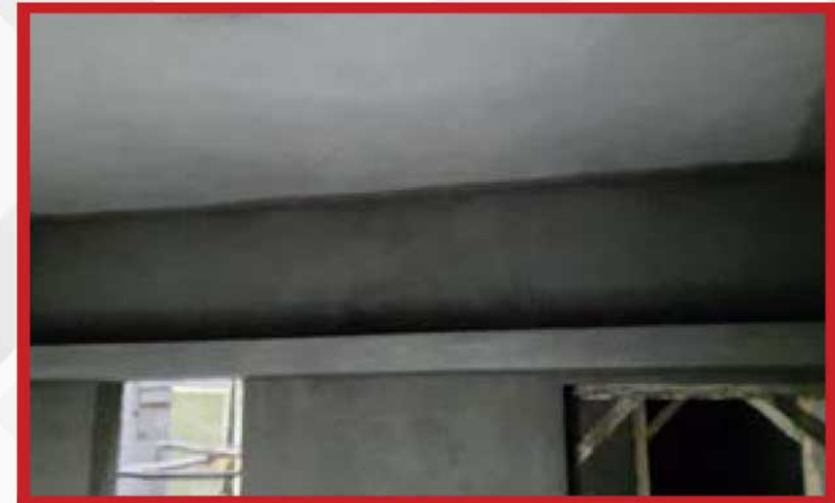
Block B - 1 st Floor: Internal plastering in progress
