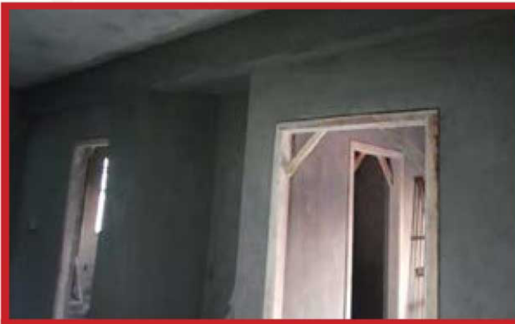
Block C - 1 st Floor: Internal wall plastering completed
