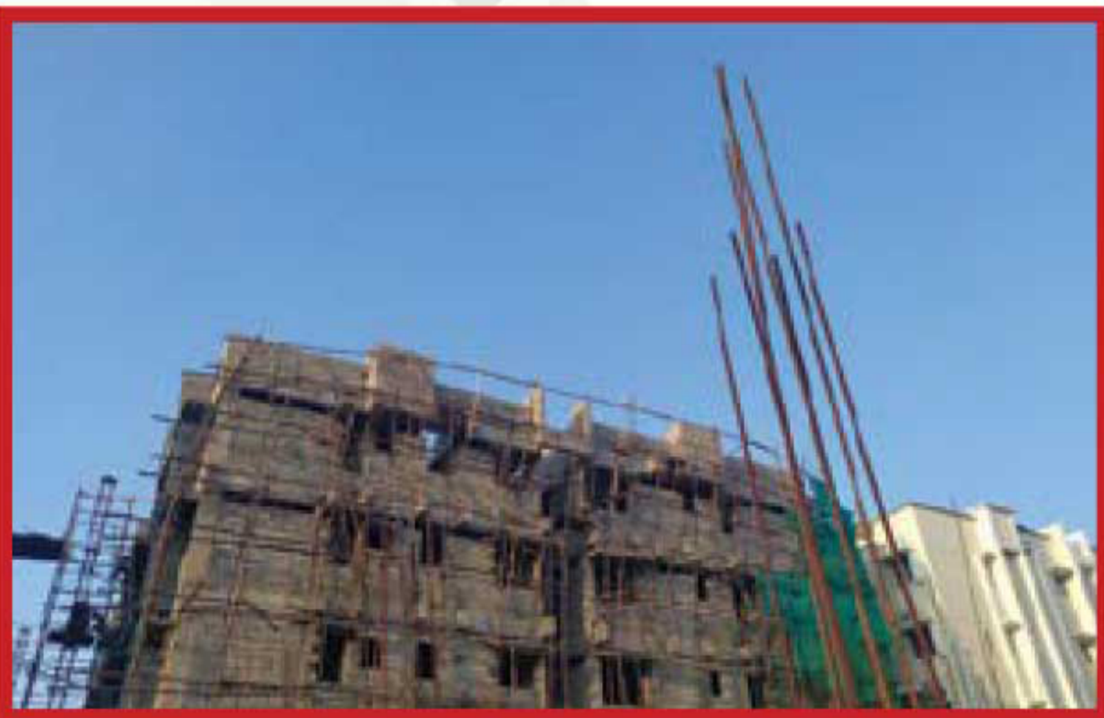
Block C - Block work in progress
